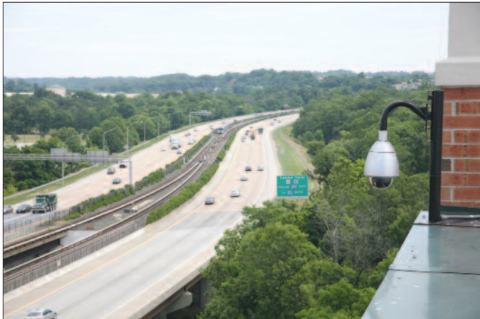
Pan-tilt-zoom dome cameras enable coverage of larger areas, providing a bird's-eye view and the ability to zoom in with precise detail.
