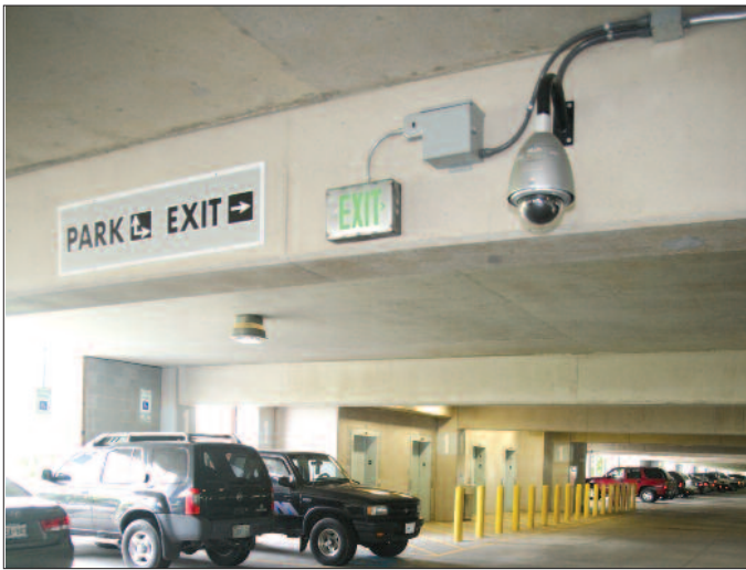
Panasonic cameras provide nearly 100 percent video coverage of the Metro Centre garage, thus exceeding a local requirement that retail parking garages be 75 percent covered by video.
