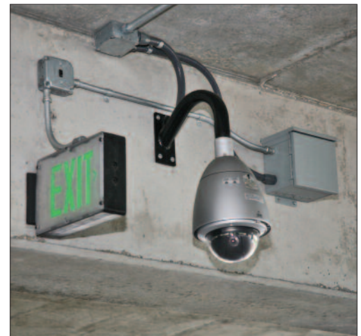
Each Panasonic all-in-one dome camera integrates a weatherproof housing, a 360-degree high-speed pan and tilt base, and a 30x optical zoom lens.
