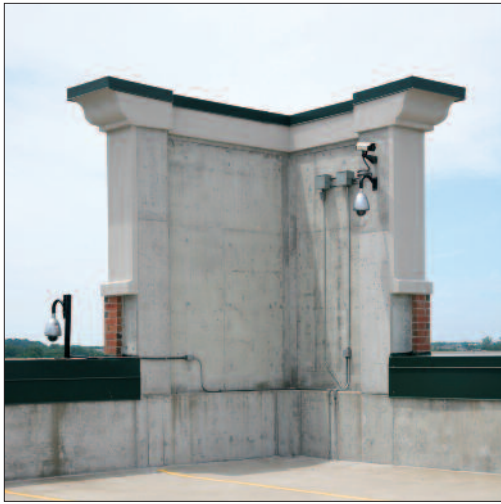
The top level of the parking garage is surveilled by Panasonic cameras which provide various views of incoming and exiting vehicles and their drivers.
